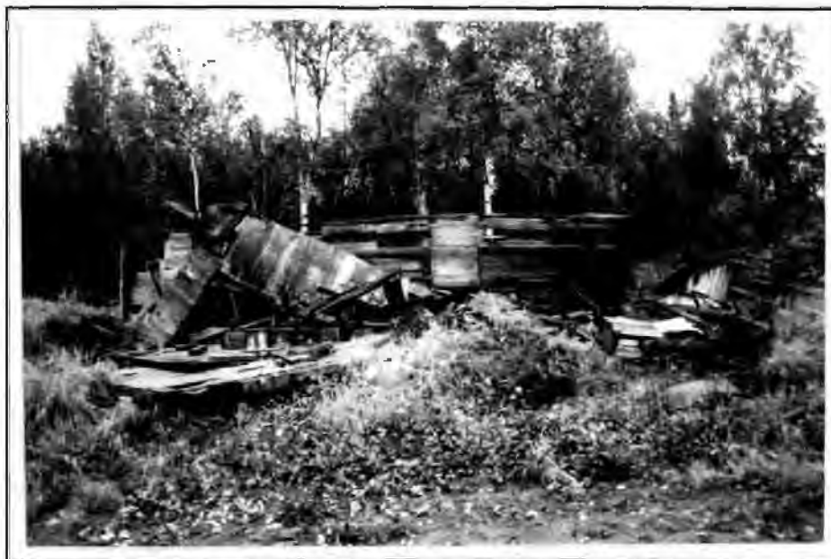
Figure 88. The Guggenheim Machine Shop, 1993. The view is looking west.
